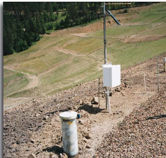
A variety of methods are available for monitoring the performance of acid rock drainage caps.
